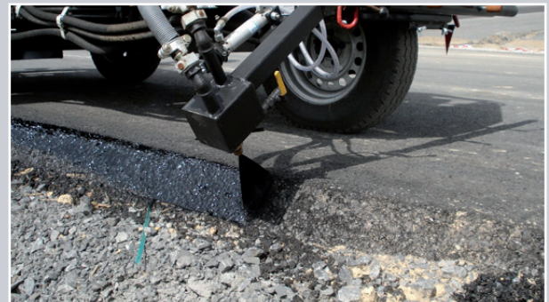
Sealing of longitudinal joints and edge with the lateral nozzle head
